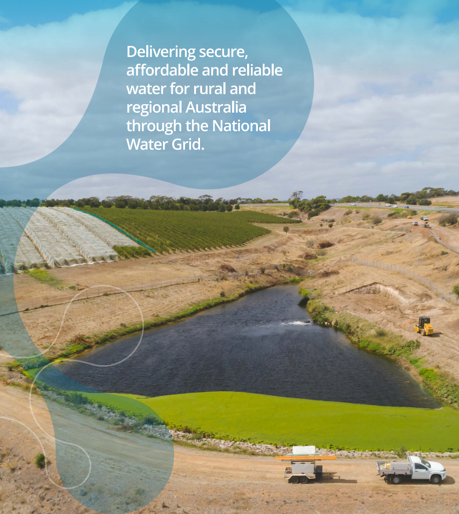
McLaren Vale Treated Water Storage, South Australia
